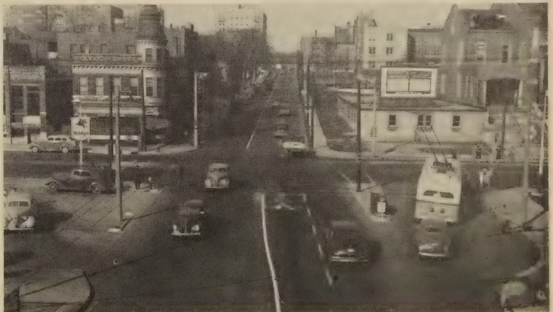
An intersection with a separated right-turning lane.
